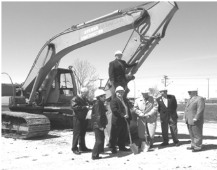
The sod turning for a new seniors housing complex sponsored by the Kivans Club took place in May. The new building will be situated west of the ANAF on Portage Avenue.
